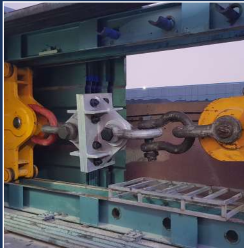
PROOF LOAD TEST OF LIFTING BRACKETS
