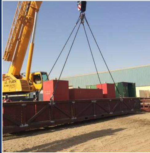
LOAD TEST OF PIPE BASKET
