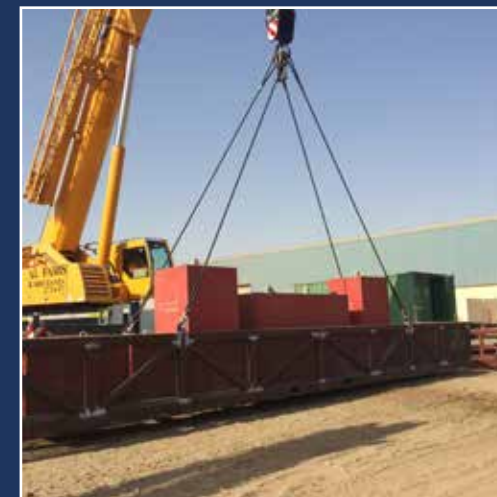
LOAD TEST OF PIPE BASKET
